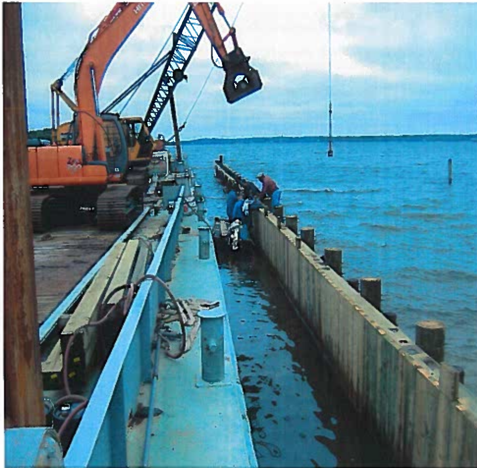
Kingston Creek Jetty, California, MD
