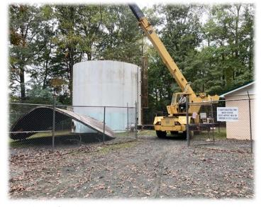
Demolition of an old ground water storage tank being completed at the St. Mary's Industrial Park water station
