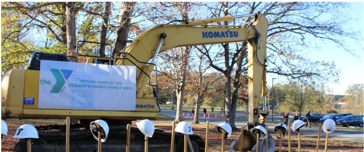
The St. Mary's County YMCA Groundbreaking
