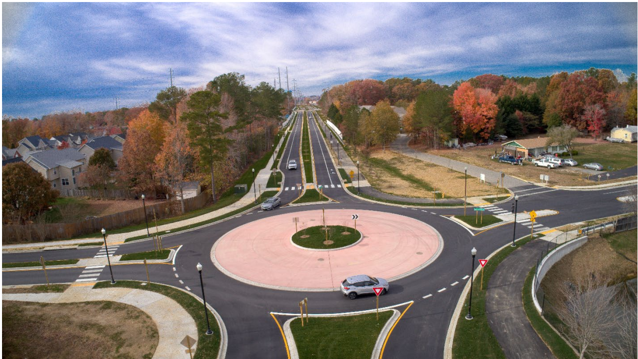
A roundabout on FDR Boulevard.
