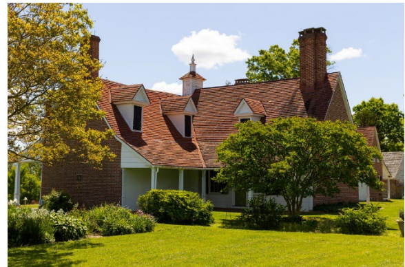
House at Historic Sotterley
