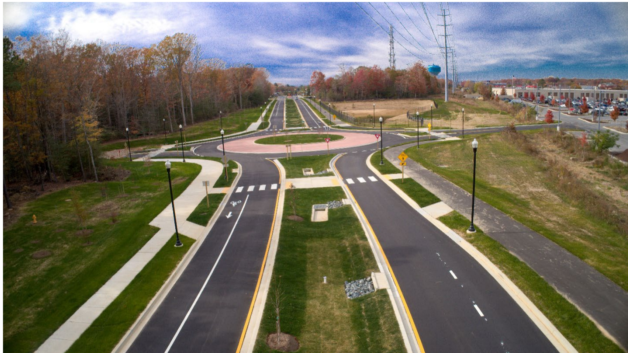
A roundabout on FDR Boulevard.
