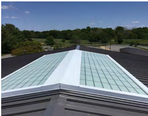
Hollywood ES HVAC & Roof Systemic Renovation
