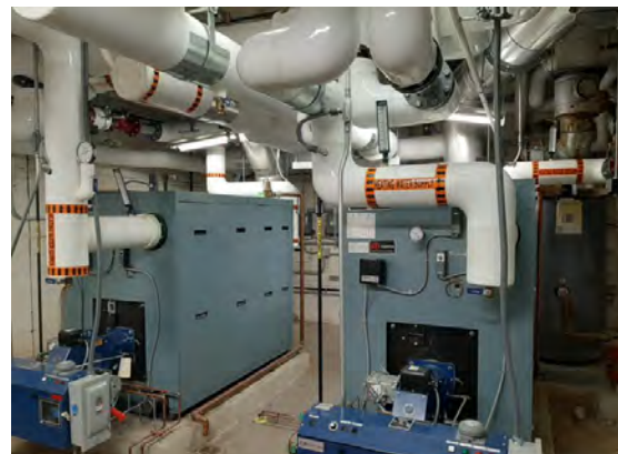
Park Hall ES HVAC & Roof Systemic
