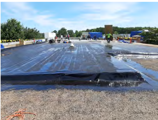
Great Mills HS Partial Roof Replacement
